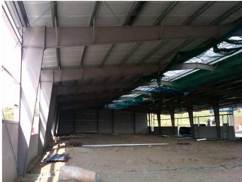
Figure 13 : Typical example of class 4 cross-section portal frame
